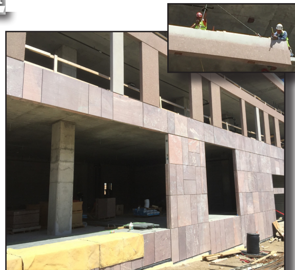
The exterior panels continue to be installed. They are now working on the south face.
